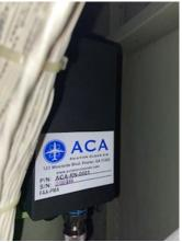
Figure 2: The ACA NPBI™ unit weighs less that one pound (right) and installs on the existing ECS output ductwork (left) to provide continuous protection from harmful pathogens.
